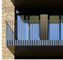
Grey Windows and Ironwork
